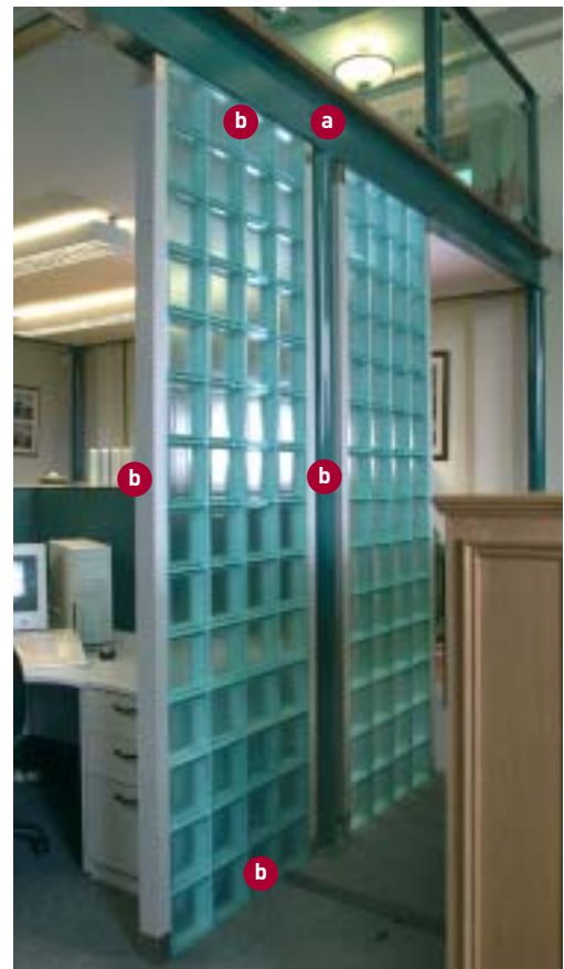
Office partitions installed using Easifix into end posts to create two vertical jambs resulting in a four sided opening.
