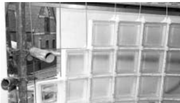
Reinforcement rods in construction
