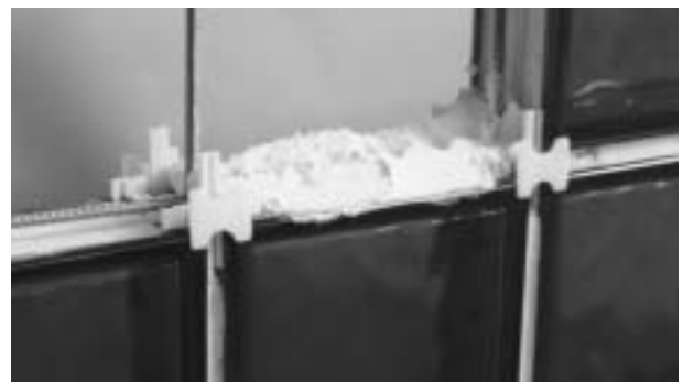
Spacer pegs and reinforcement rods
